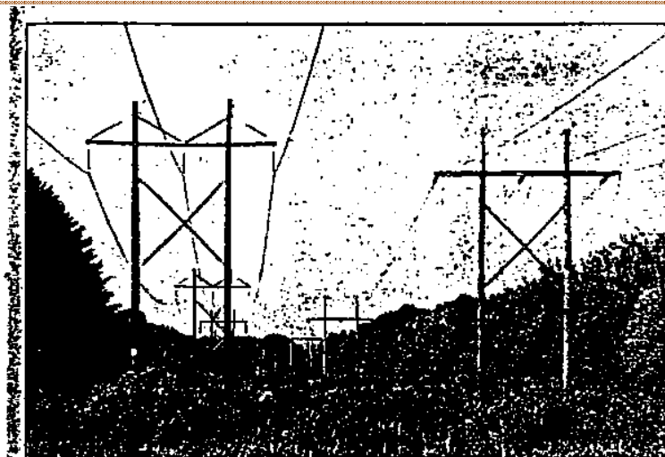
Figure 12 Higher wood structures, supporting heavier conductors, are built alongside existing line, which is later removed
